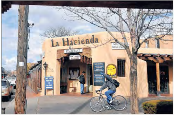
La Hacienda restaurant, a fixture on the Old Town Plaza for about 60 years, is closing its doors today, but owner Ted Garcia says he's trying to work out some matters with the building's landlord over electrical and other issues.
